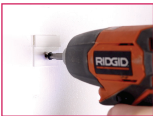
Drill screws through corner pieces or mounting brackets into wall studs
