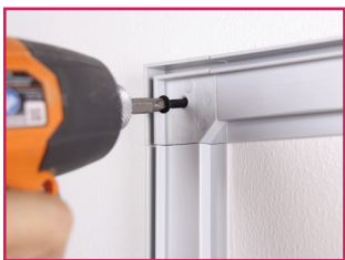
Drill screws through corner pieces or mounting brackets into wall studs
